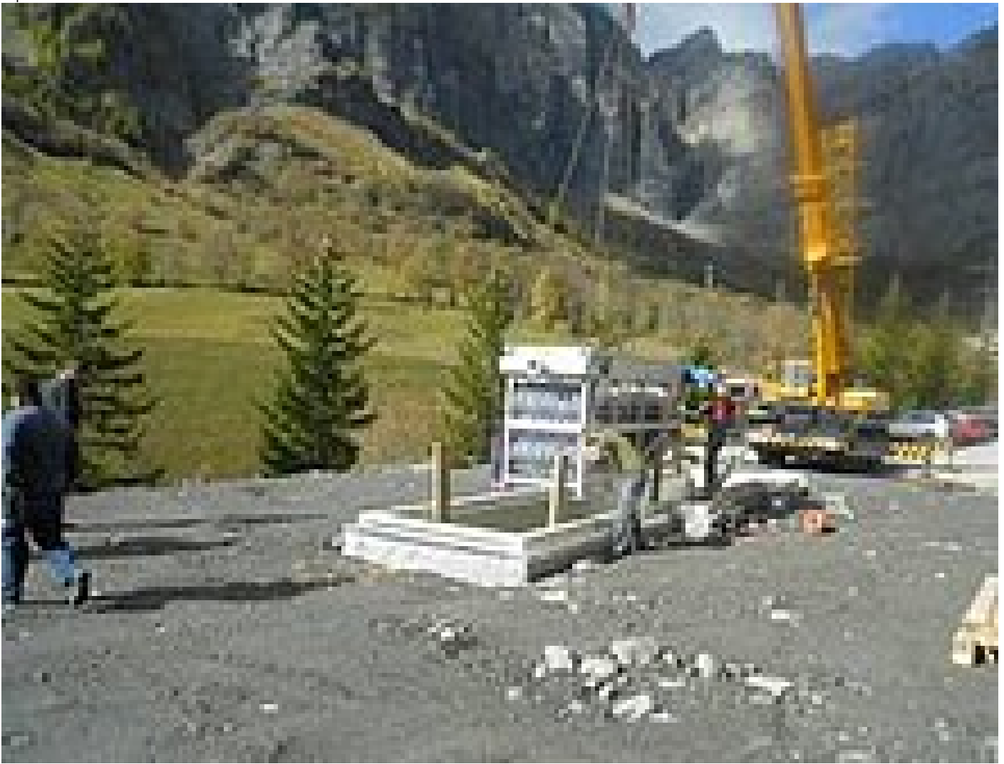
HUBER RoWin Heat Exchanger (tank version) during installation
