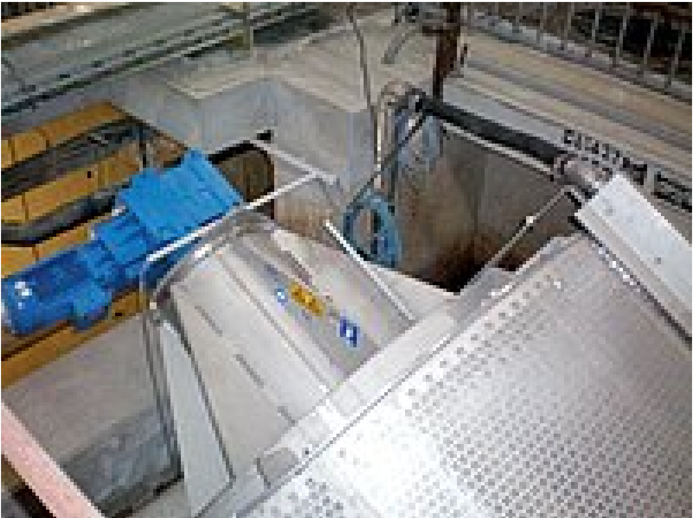
RoMem liquid fine screen with apertures up to as small as 0.2 mm
