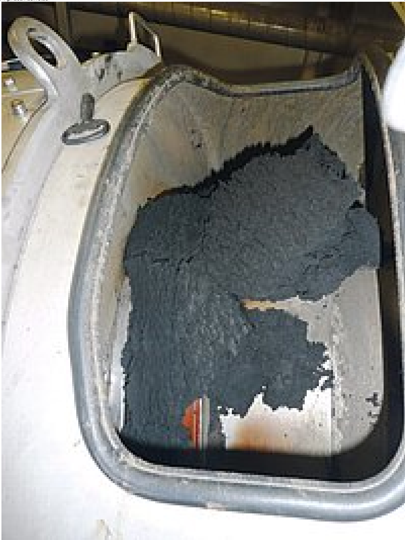
Dewatered sewage sludge from the RoS 3Q 620 screw press
