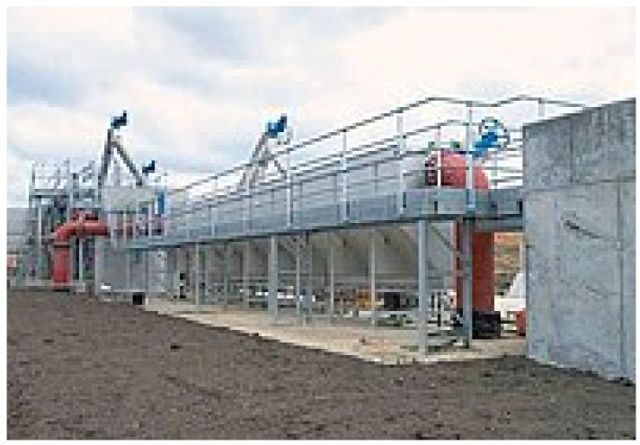
Longitudinal grit trap with grit removal screw
