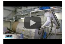
Video: HUBER ROTAMAT® Wash Drum RoSF9 in a grit treatment process for coarse material separation
