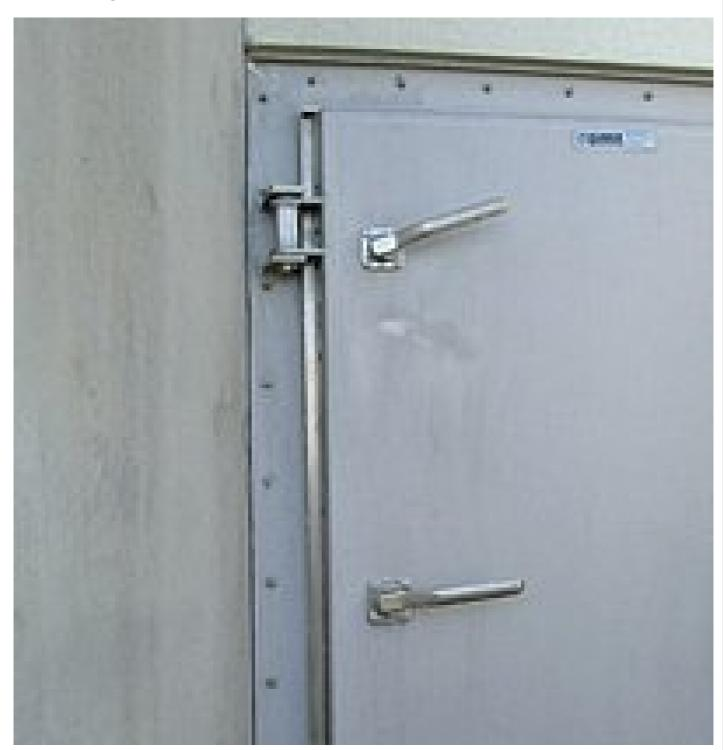
Access door for the field of potable water supply, especially in areas where flooding is likely. Flood-proof up to 2m water head.
