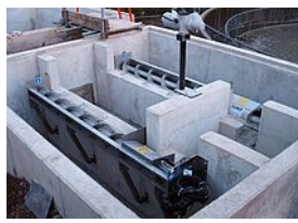
HUBER Storm Screen ROTAMAT® RoK1 TS with a cross conveyor for high solids loads
