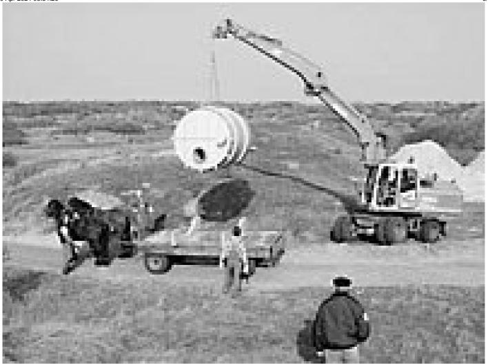
Water supply of the North Sea Island Baltrum is via a pipeline system from the main land and five wells are provided for emergency cases. The wells were established in 1960 and have brick shutoff structures. While the inspection of the buildings showed the proper function of the wells, there has been a complaint about the brick structures from the hygienic and constructional view. Repair of the old buildings rejected for cost reasons.
