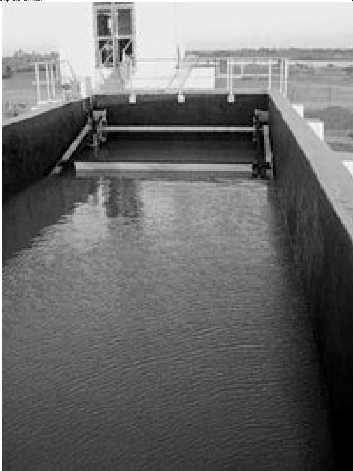
Filled sedimentation tank
