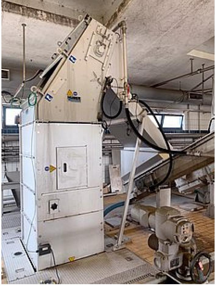
The photo shows the HUBER Multi-Rake Bar Screen RakeMax® CF, which combines the advantages of the proven RakeMax® with the positive features of a centre flow screen, installed on a size 5 wastewater treatment plant.
