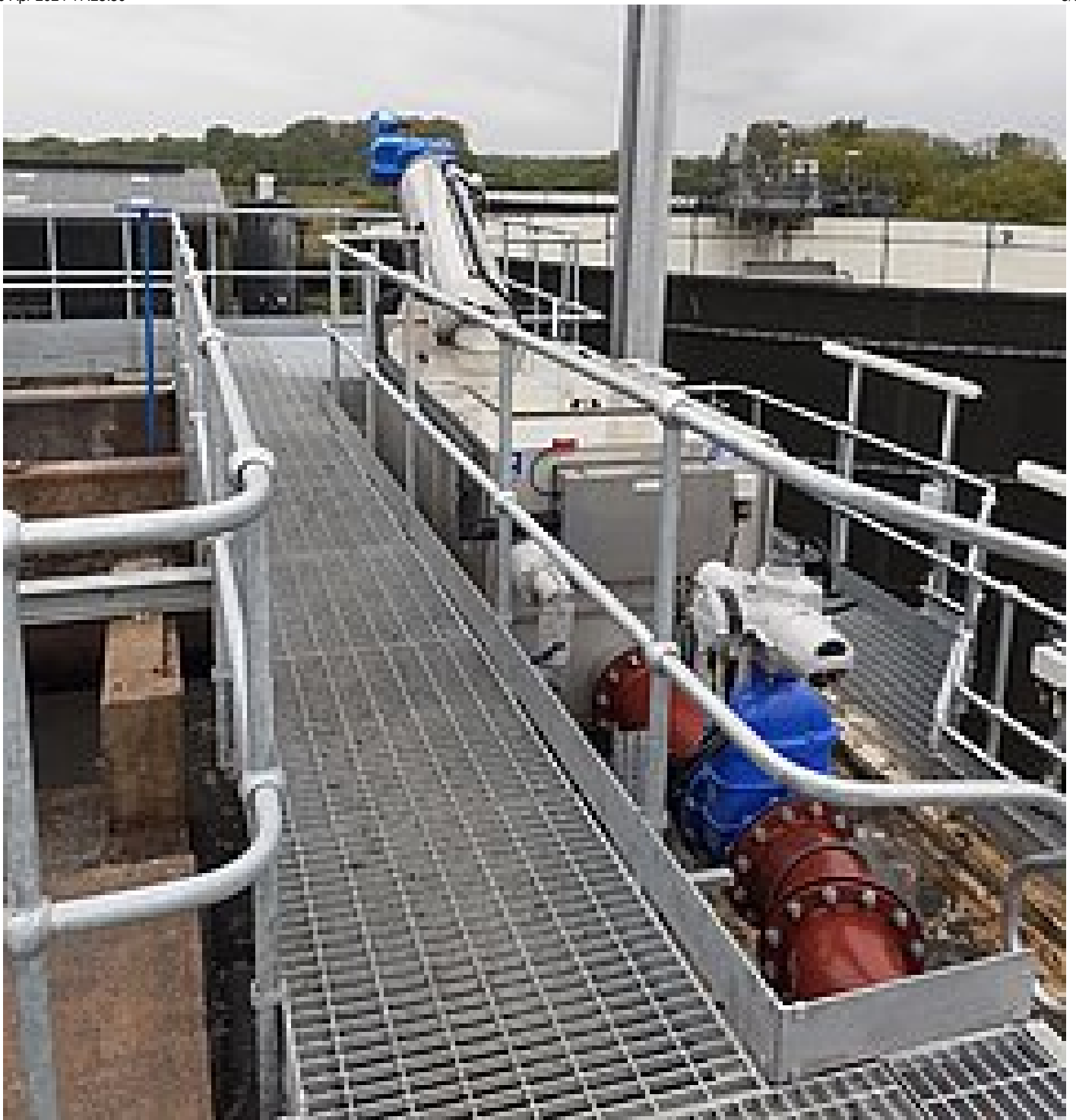
New screen adjacent to the old channel
