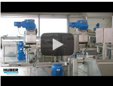
Video: HUBER Membrane Screen ROTAMAT® RoMem - here at a municipal WWTP https://www.youtube.com/watch?v=YsFSSEnSAMs
