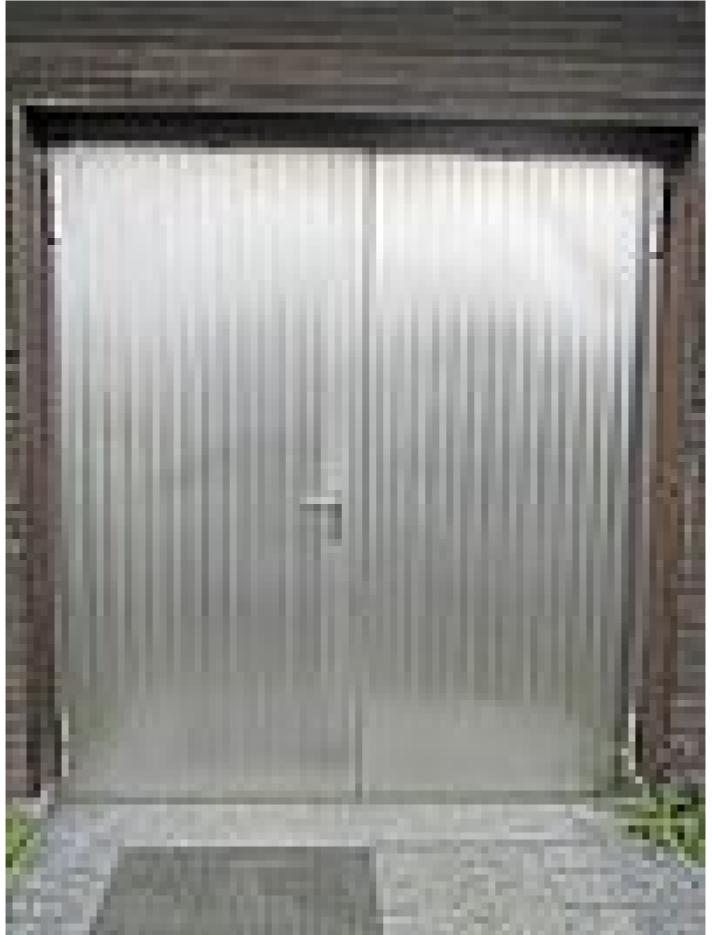
The door leaves and frame closing flush, the fixable and swing leaf opening to the outside (in escape direction).
